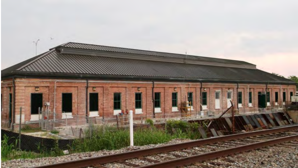
Fig. 2 Overall view of typical Drainage Pump Station. Pump Station 7 is shown here.
