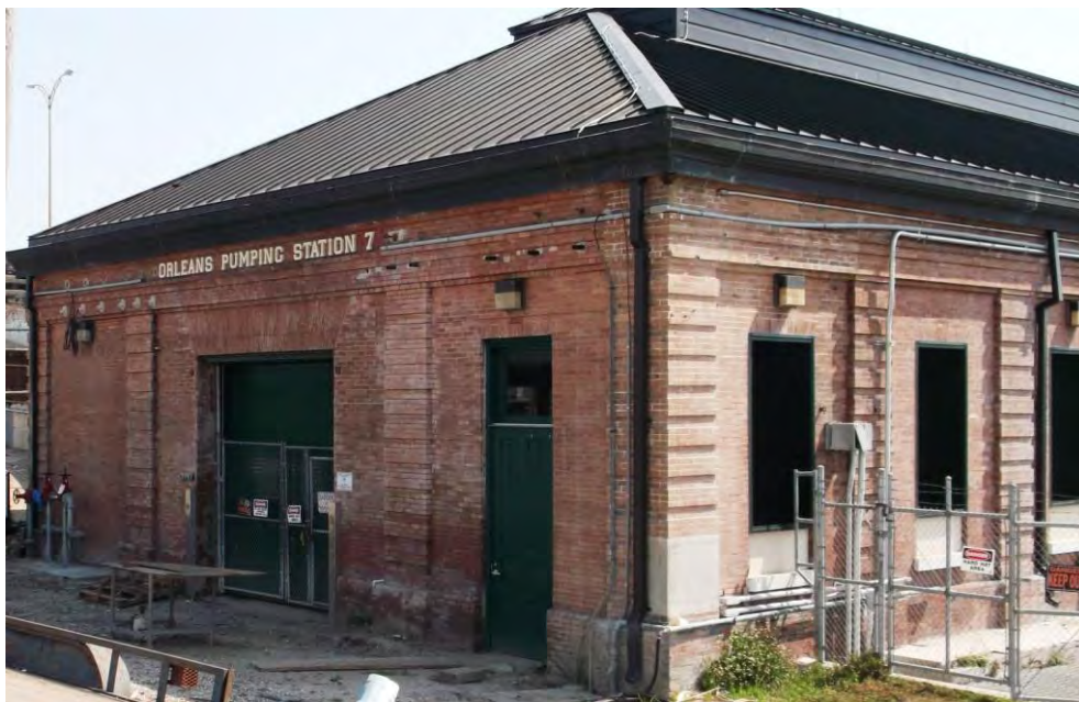
Fig. 9 Overall view of southwest corner of Drainage Pump Station Number 7 showing the clay brick masonry exterior walls after completion of the strengthening project.
