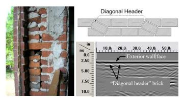
Fig. 2 Walls were built of poor quality construction (left) with many internal voids. Surface penetrating radar was used to locate voids and also identify hidden header locations. Hidden "diagonal" headers were missing at many locations, requiring remedial tie installation. The radar trace at lower right shows strong reflections at each header brick location.
