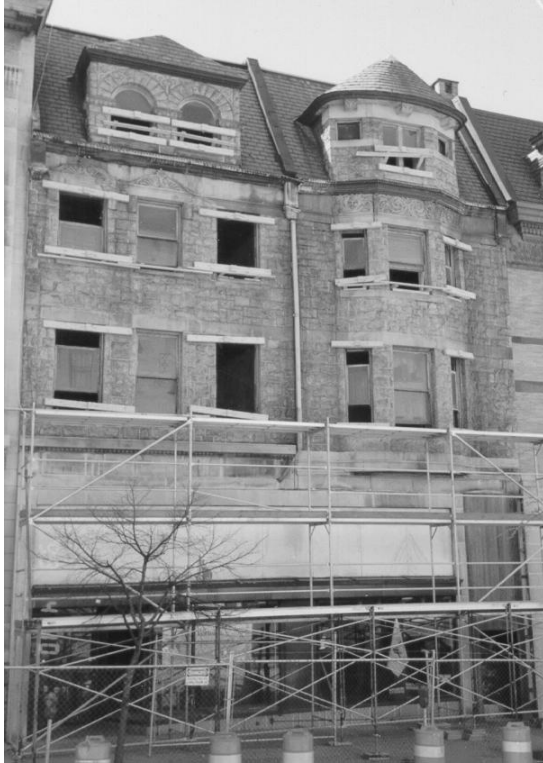
Figure 1. Street elevation of the building, showing the façade before stabilization.
